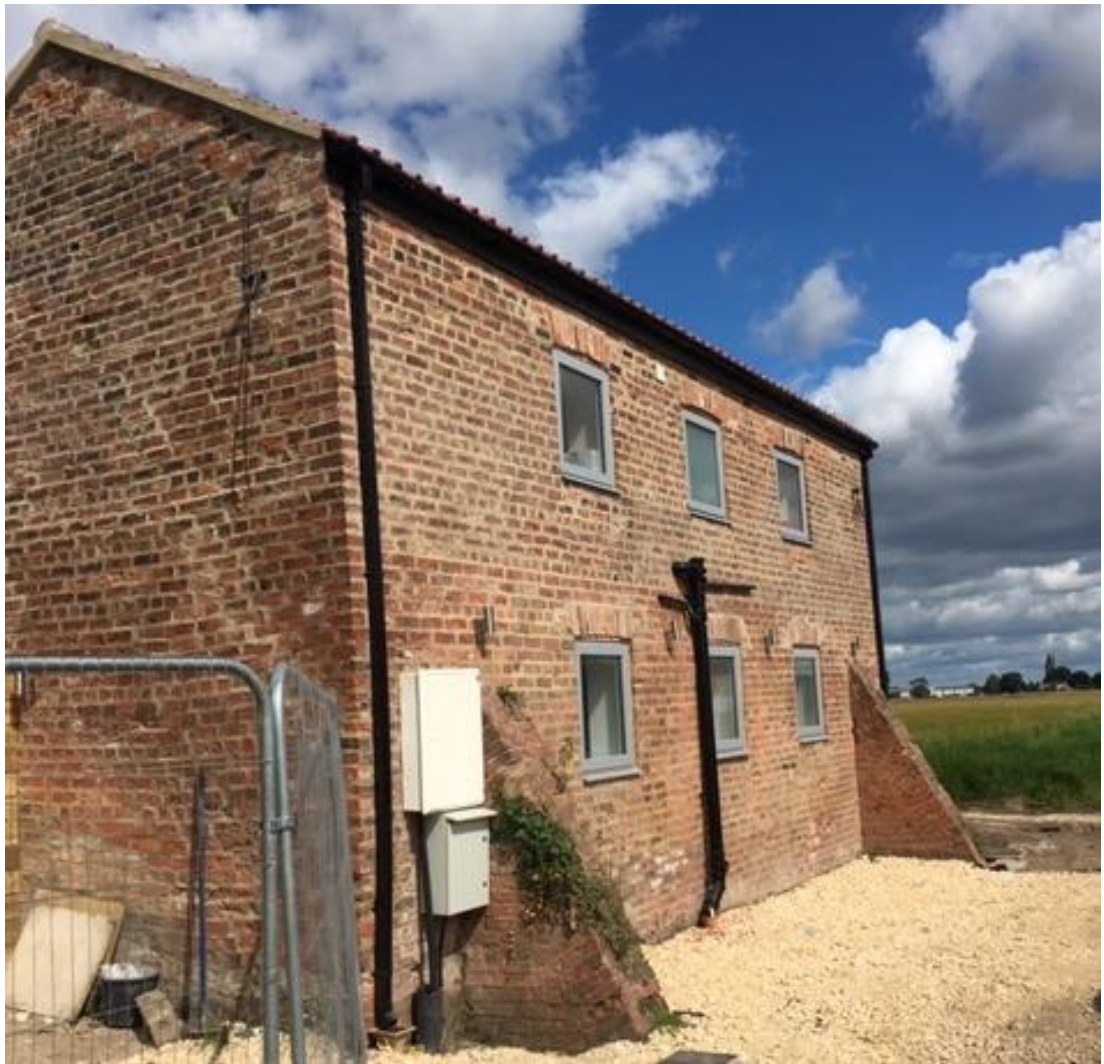
View of the east elevation
