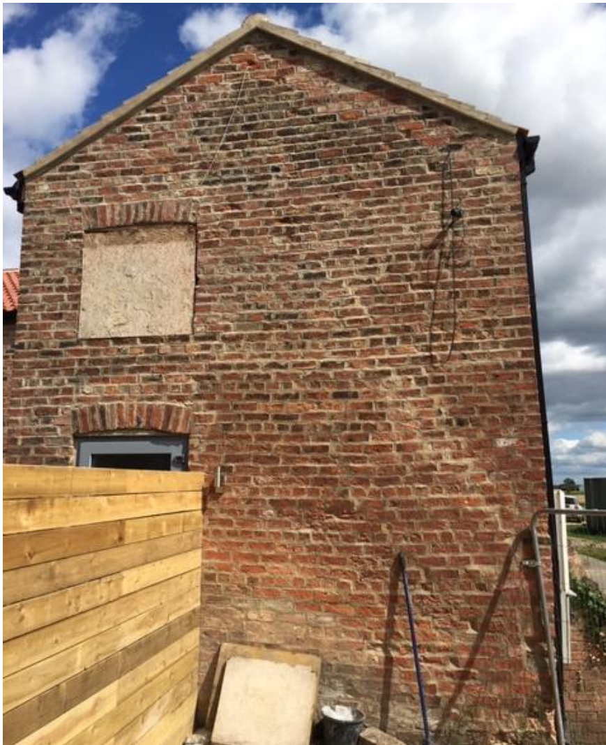
View of the south and west elevation
