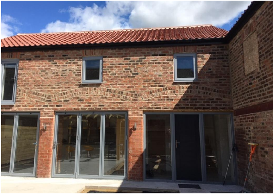
View of the south and west elevations
